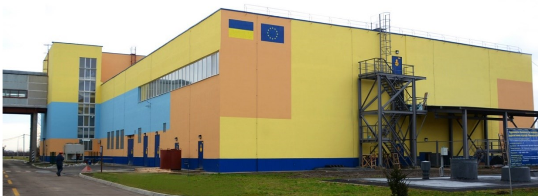
Figure 2.9. Exterior of CRWP building
