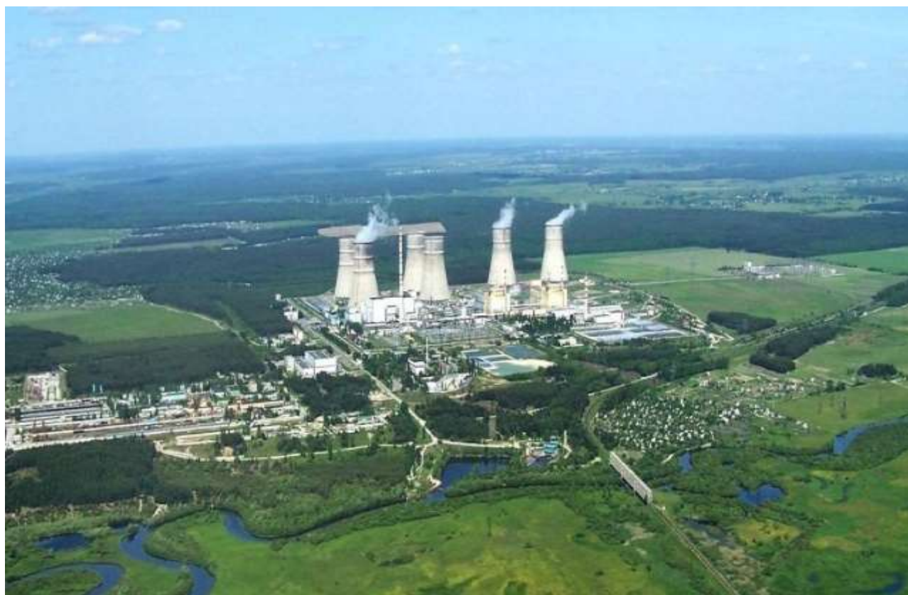
Fig.1.1 a) General view of Rivne NPP site
