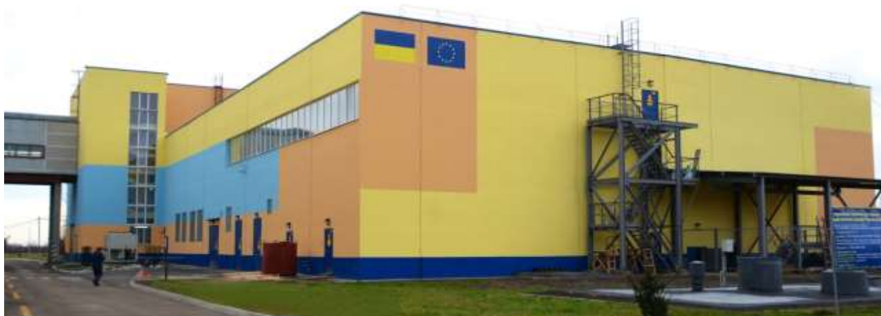
Fig.2.5. Exterior of CRWP building
