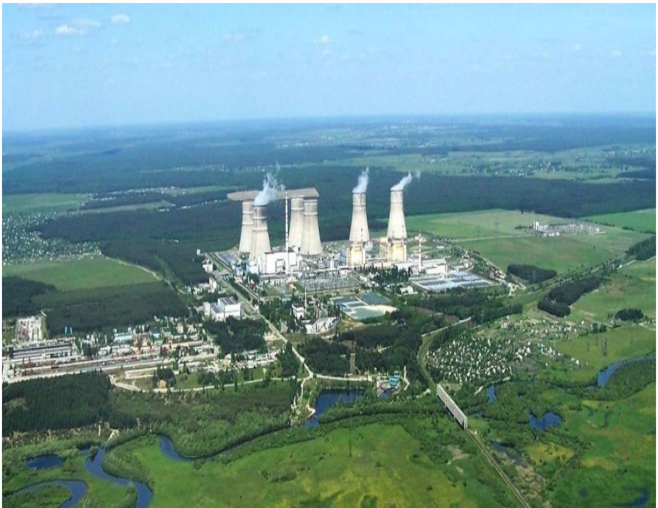
Figure 2.1. General view of Rivne NPP site
